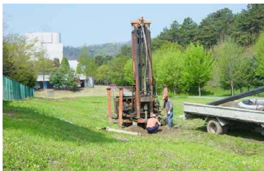
Figure 3: Drilling on the KEPRI site in April 2003 (photo Choi)
