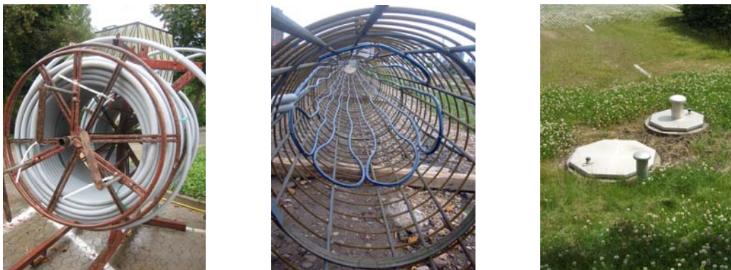
Figure 2 Coil with borehole heat exchanger pipes (left), energy pile / foundation pile (middle) and well [source: IGS, TU Darmstadt and IEK University Hannover]
