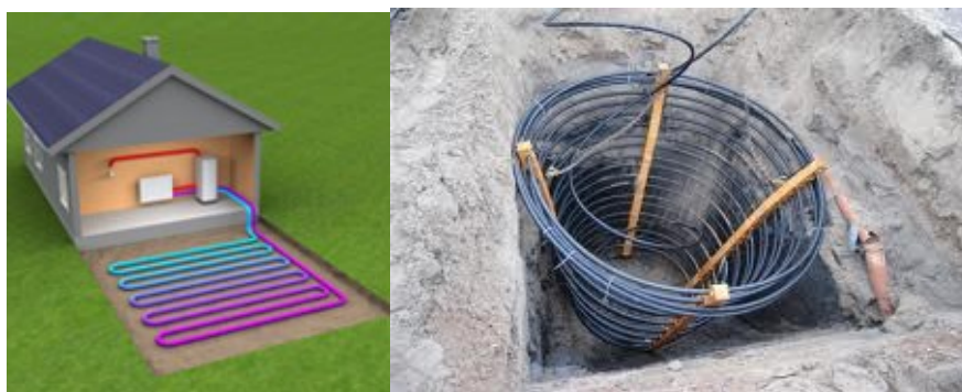
Fig. 8: Very shallow CLOSED LOOP SYSTEMS (Left: horizontal closed loops, Right: basket system)
